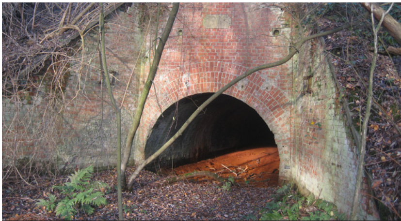
Tunnel 36, foto PA
